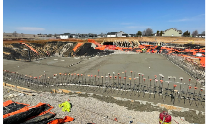
Lap pool floor poured
