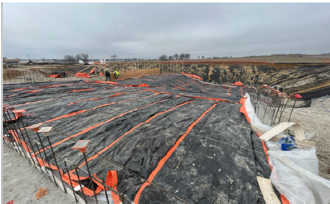
Lap pool floor covered
