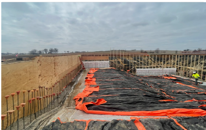
Lap pool wall forms being installed
