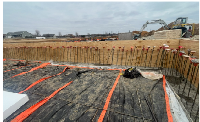
Lap pool wall forms being installed in the shallow end
