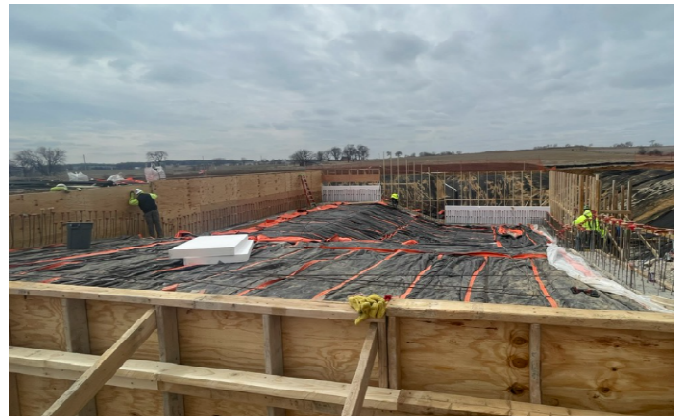
Lap pool wall forms being installed
